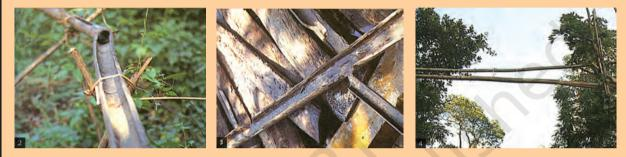
**Picture 2 and 3:** The channel sections, made of bamboo, divert water to the plant site where it is distributed into branches, again made and laid out with different forms of bamboo pipes. The flow of water into the pipes is controlled by manipulating the pipe positions.
