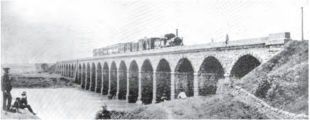
Fig. 1.4 First Railway Bridge linking Bombay with Thane, 1854
